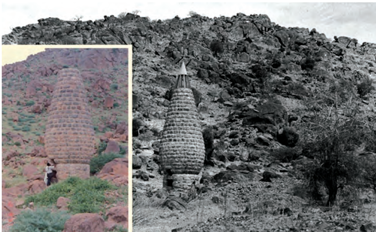
Figure 13 - Stone incinerators built by Wellcome in Jebel Moya camp for waste disposal. Box: A more recent photograph of the stone incinerator.
