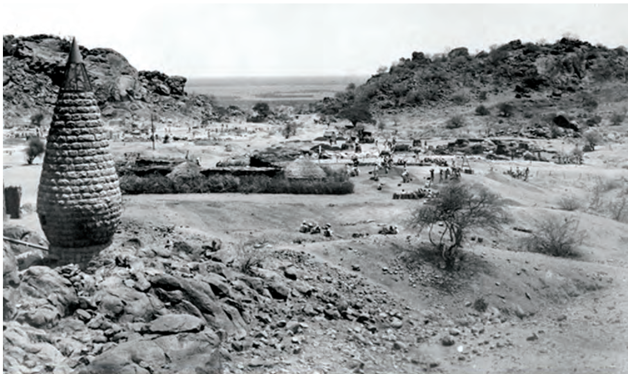
Figure 12 - Stone incinerators built by Wellcome in Jebel Moya camp for waste disposal.
